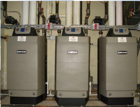
High Efficiency Boiler Installations
