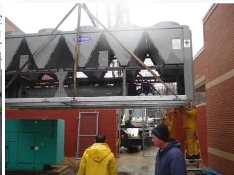
Air Cooled Chiller Installation
