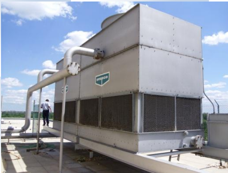
Cooling Tower Installation and Repairs
