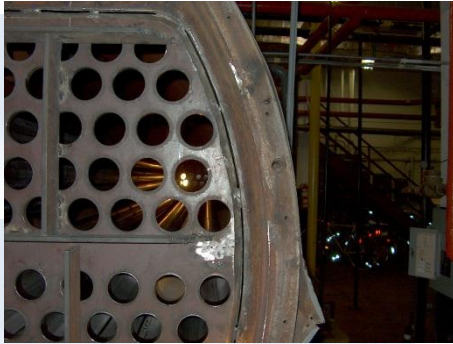
R-1 Welding Repairs
